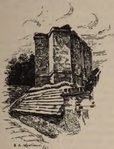
Stack of chimneys in Nell Gwynn's house from which the coin was taken
